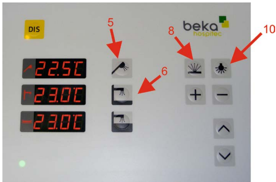
Figure 22: Check the outlet temperature with the external thermometer! The process is now complete.
