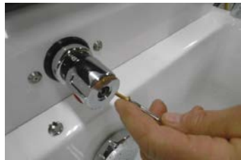
Figure 19: Install the rotary knob with the cross bolt
