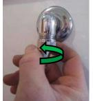
Picture 4: The picture shows the shower hose unscrewed from the elbow fitting
