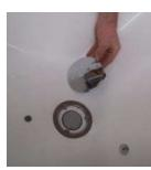
Picture 4: The rotary actuation must be positioned horizontally (Viega logo must be recognizable) before
